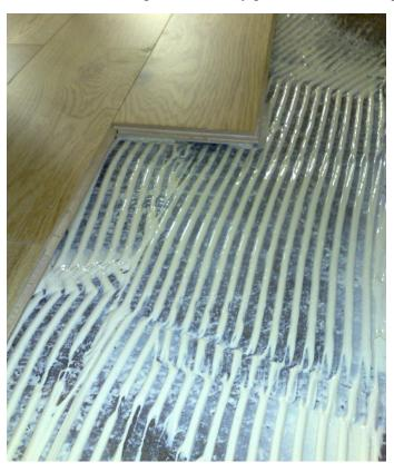
The image on the left is the correct application of the SW890 adhesive.
