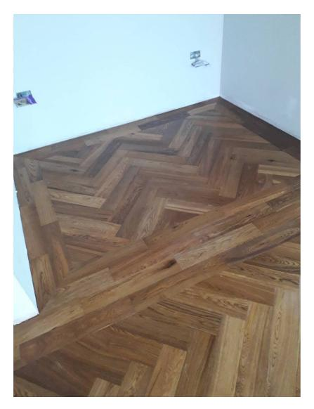
The image to the left shows how the same herringbone parquet blocks can be used to create a border and different areas in a room.
