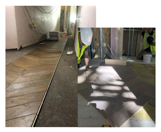
Whichever method is used, the crown line must be perfectly straight and in the centre of a room. For chevron it can be in the centre of a doorway entrance, or other "vista" where the eye will be drawn to.
