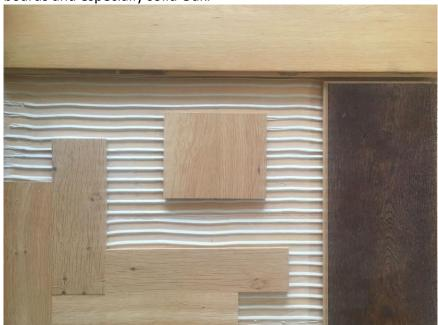
The image to the left shows how the adhesive should be applied. You must always use the correct trowel which is dictated by the board and subfloor.
