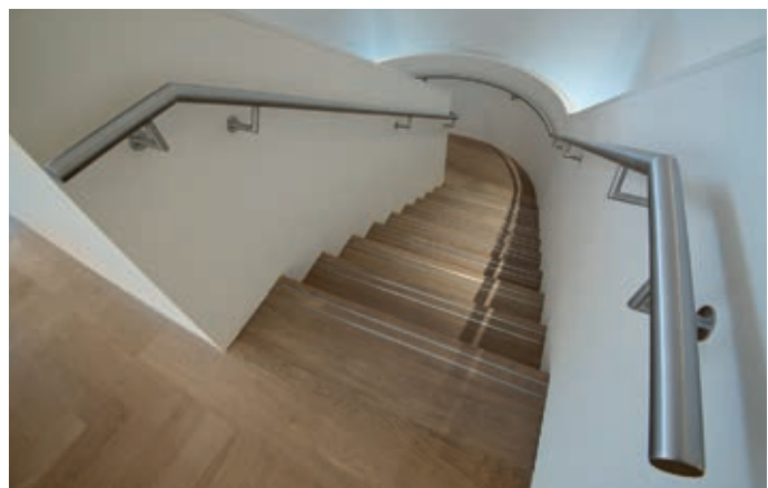
Stairs clad with light fumed boards to match the E212
