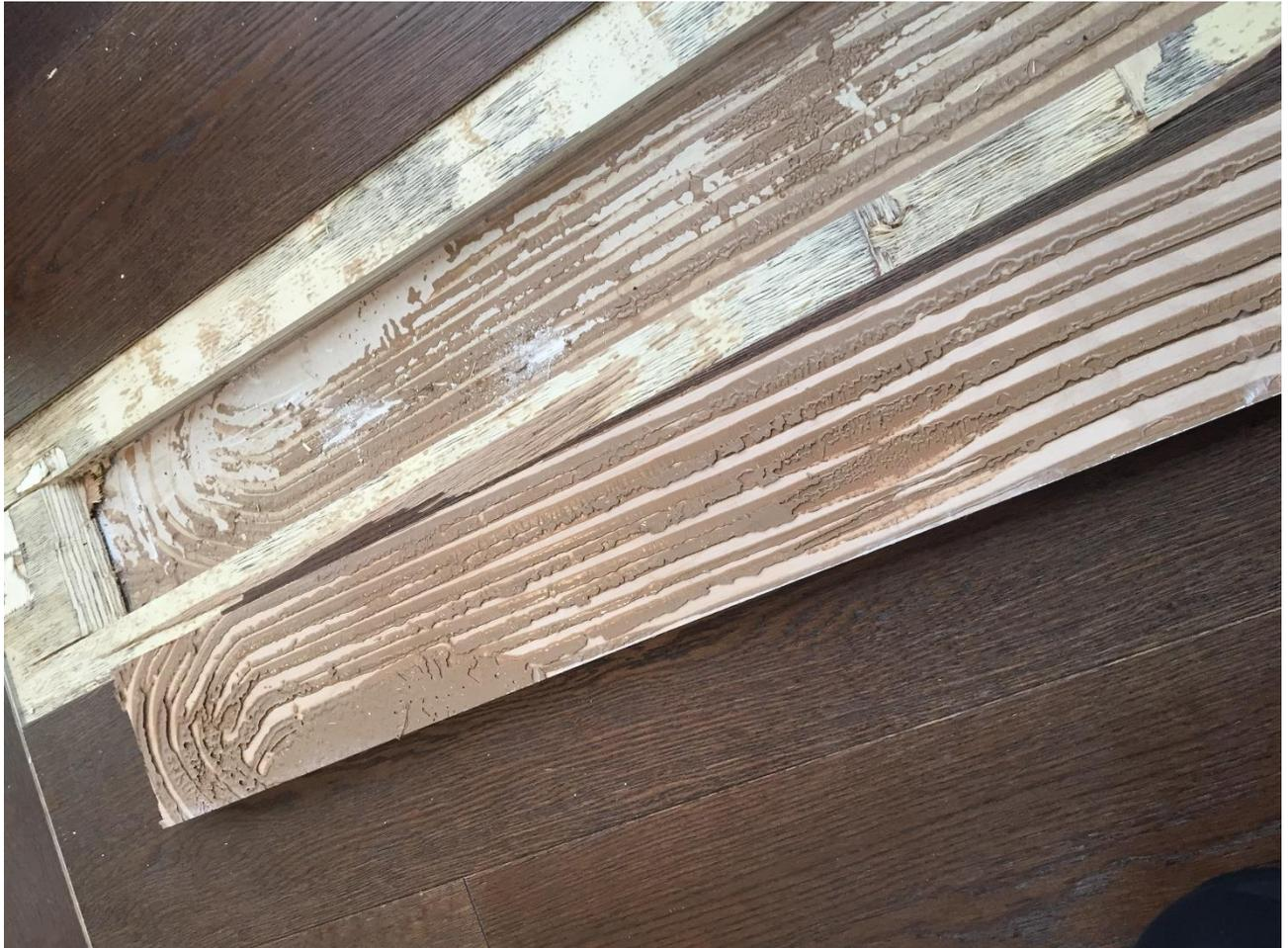
The image above shows what happens to wood flooring when the laitance is not removed. As you can see there was a lot of moisture left in the screed and then the board was lifted it shows that some of the Laitance came away (white powder type) as the adhesive could not bond properly and there was a hollow sound when tapping the board.
