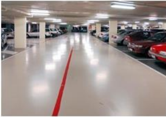
Figure 5: Coating used to protect surface, delineate areas and facilitate maintenance
