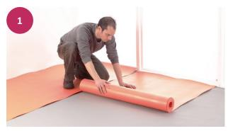
Ensure subfloor is clean and flat\*. Unroll at a 90° angle to the direction of the WOOD floor, covering the area to be laid. To assist laying, apply double-sided tape to the perimeter of the sub-floor. If laid on a concrete sub-floor the SW-633 can be used as a vapour barrier. This is not a Damp Proof Membrane.
