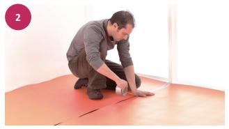
The first row should be laid with a minimum of 20mm up the walls. Butt the next row edge tightly to the first, ensuring that they do not overlap. Carefully tape the joints using a water proof tape. All rows, including the last, should also be laid with a minimum of 20mm up the wall if using a trim or scotia.
