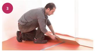
It is better to put the underlay and wood flooring under the skirting and as the underlay is only 2mm and the flooring 15mm or 20mm it is easy to cut the bottom of the skirtings if they are already installed. If you have new skirting boards, fix after the installation of the flooring and lay the SW-633 right up to the wall. Lay the flooring on top of the SW-633 referring to The Solid Wood Flooring's instructions.
