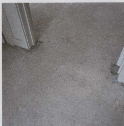
Above: Builder's screed is rarely smooth enough for vinyl flooring
